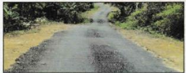
Rural Road, Tripura
